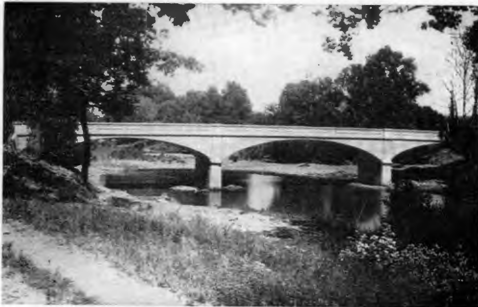
ELKINS BRIDGE OVER WHITE RIVER, WASHINGTON COUNTY, ARKANSAS
