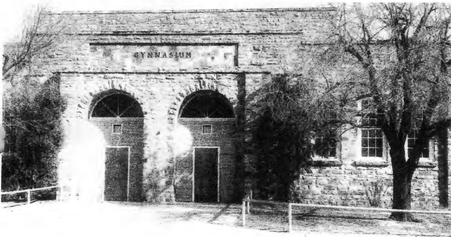
Greenwood Gymnasium with the front entry alterations, circa 1960.
