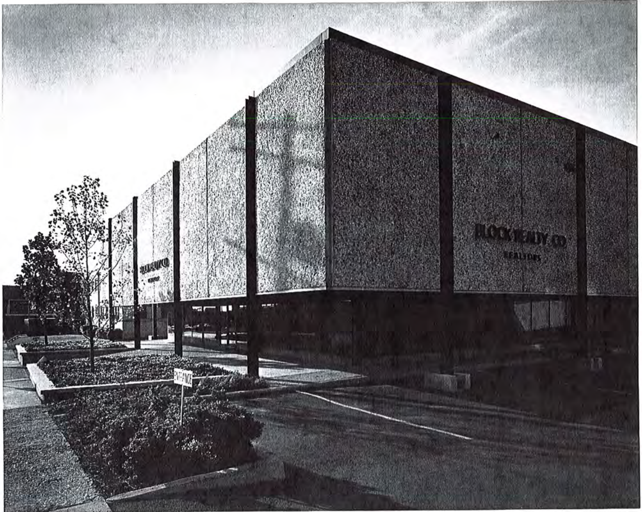
Figure 3: North and west façades of the Block Realty Building, looking southeast, 1965.
