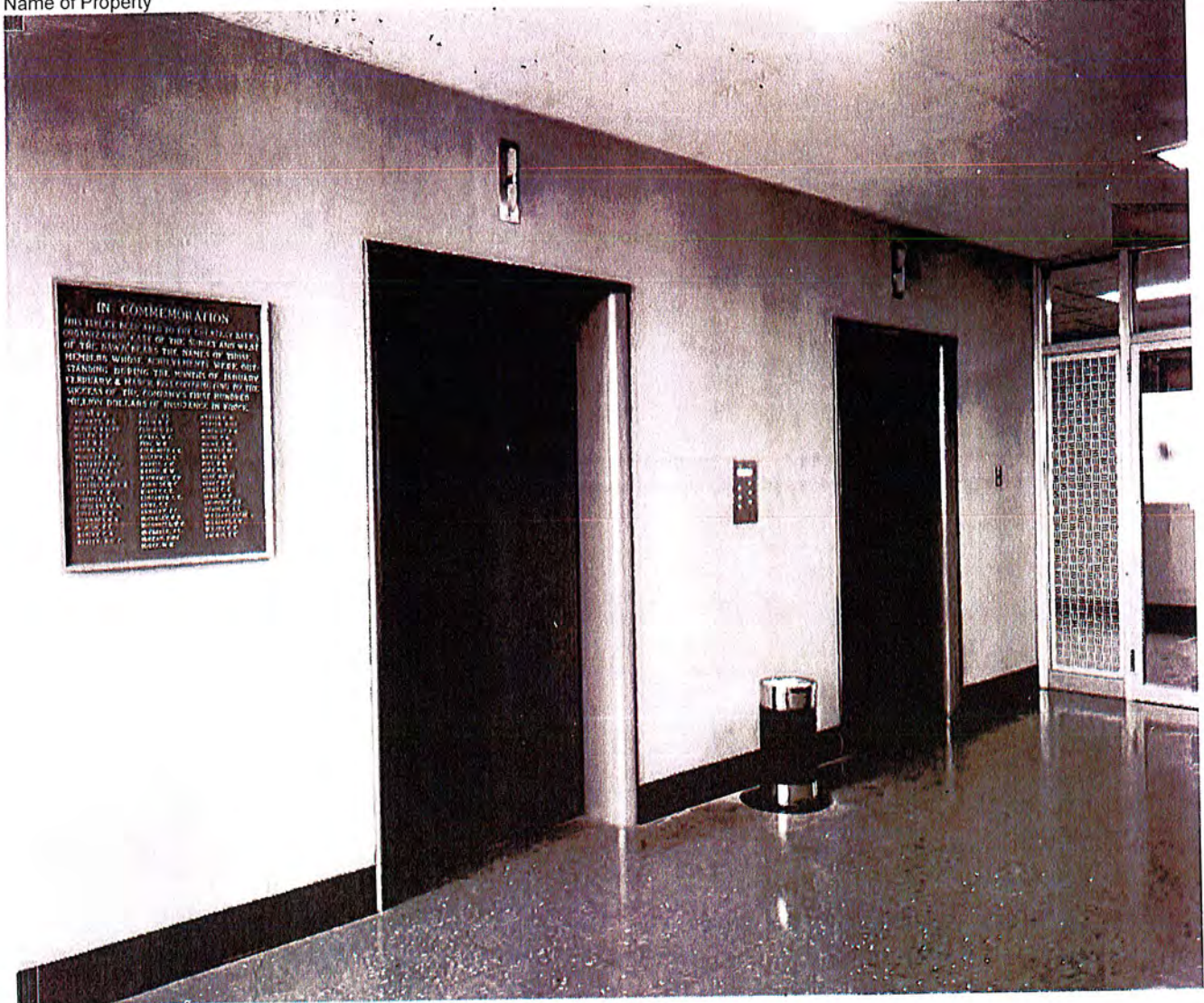
Fig. 5 – First floor elevator lobby
