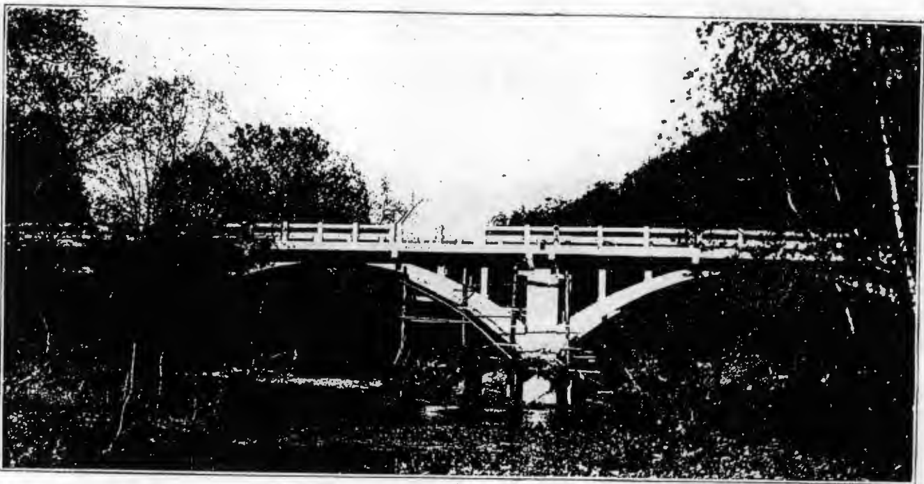
A pretty view of a Concrete Arch Bridge under construction over War Eagle Creek east of Huntsville in Madison County. State Highway No. 68.
