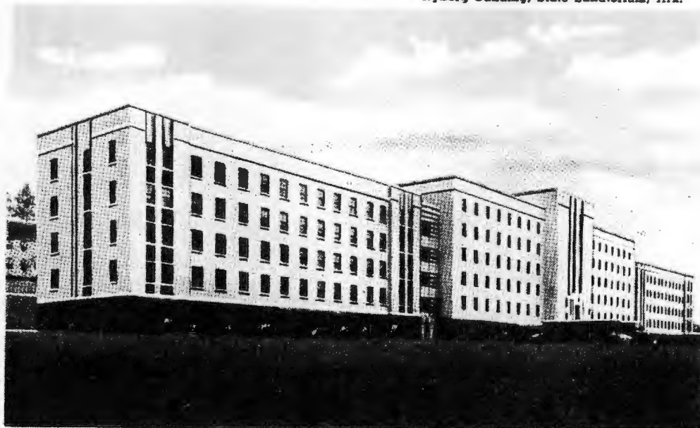
Nyberg Building, State Sanatorium, Ark.
