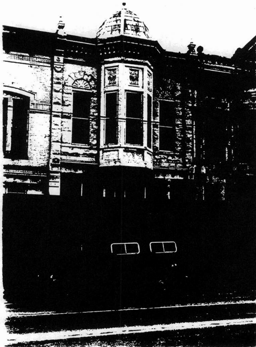
HS-46 Stitt Bldg. 516 Central Hot Springs Central Ave. Historic District A. Jones & J. Vosmik-photographers March, 1984 Negatives at AHPP Viewed from the Northeast CONTRIBUTING
