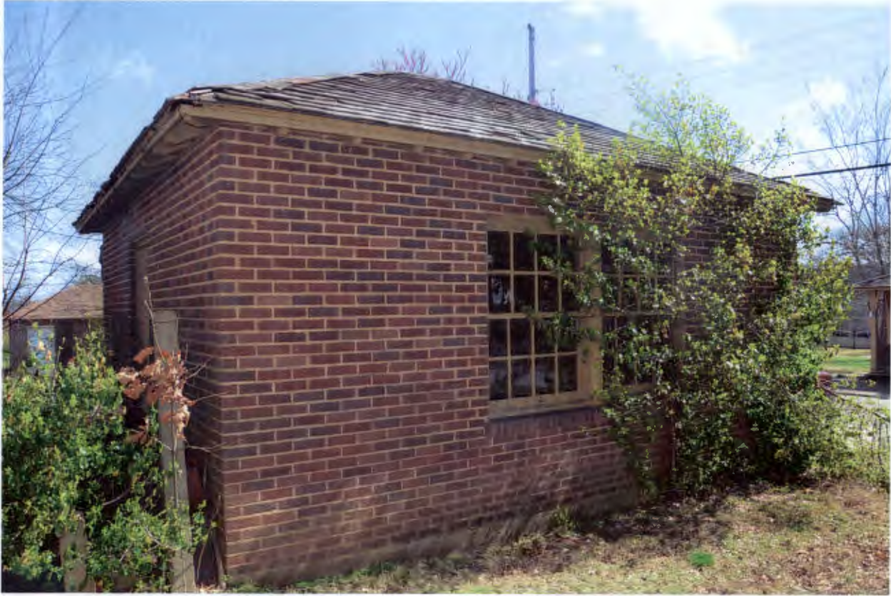
Figure 2: Garage of the V. C. Kays House, looking southeast, 2012.
