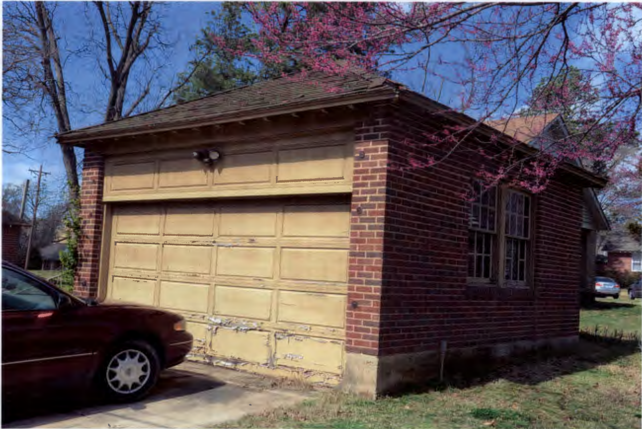
Figure 1: Garage of the V. C. Kays House, looking northwest, 2012.
