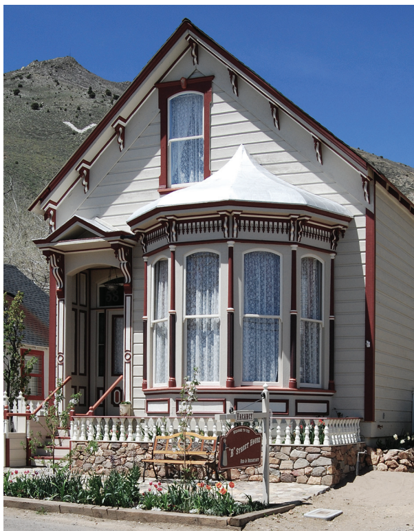
58 B Street, Virginia City, Nevada (1875). Rehabilitated as a bed and breakfast. Courtesy Chris Eichin.
